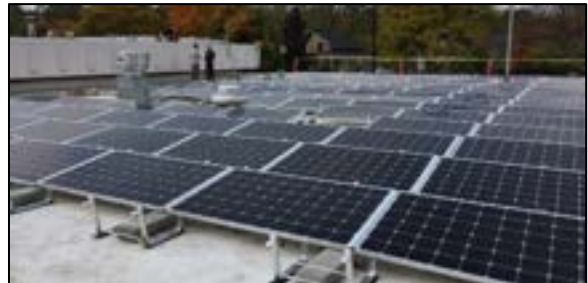
Figure 2. Solar array Installation on City of Ypsilanti Fire Station. Source: solarypsi.org
